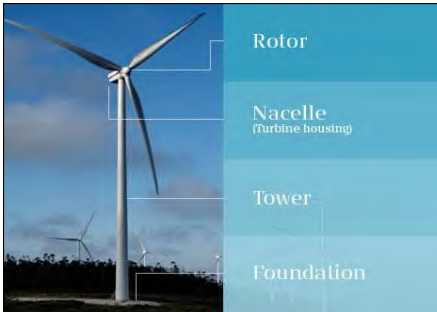
Plate 4-1 Wind turbine components
