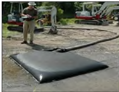
Plate 4-5 Silt Bag with water being pumped through
